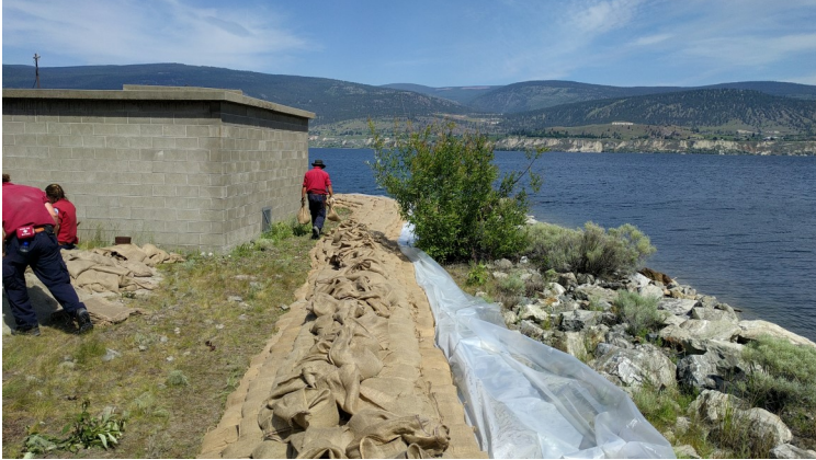
Sandbagging around the Lake Pump Station
