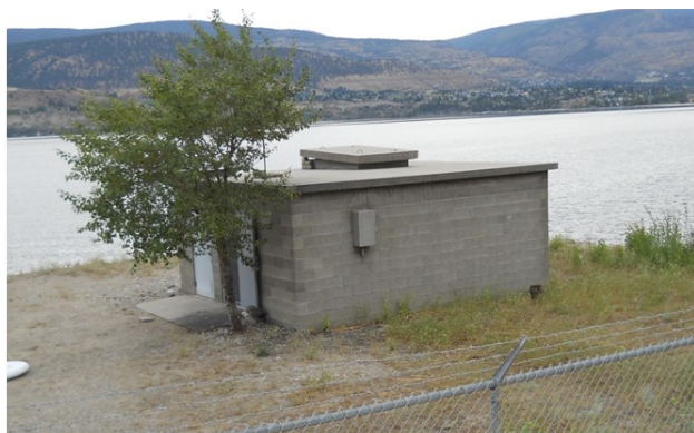
Lake Pump Station on Hwy 97
