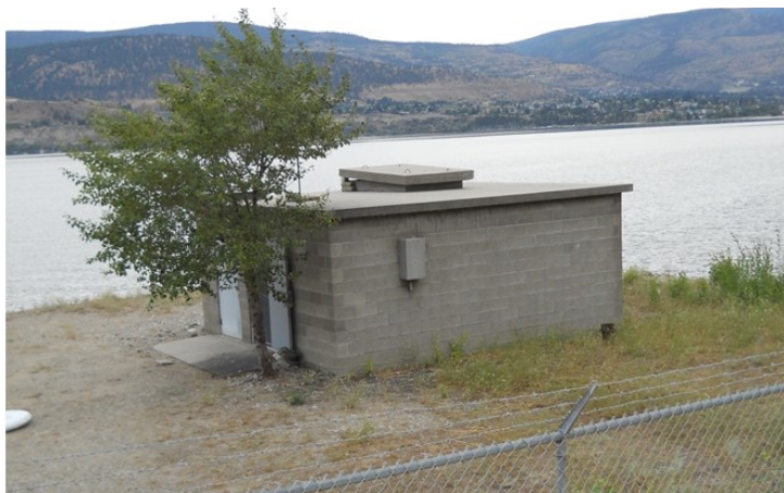
Lake Pump Station on Hwy 97
