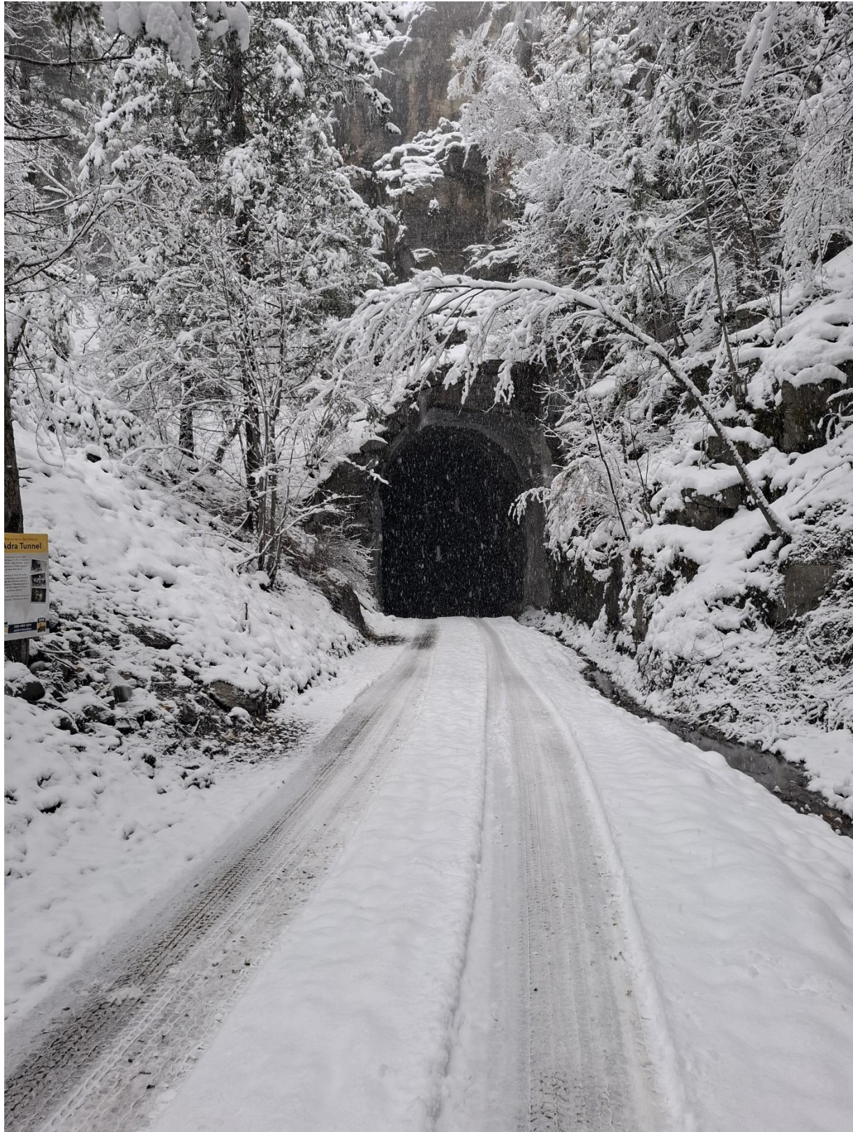
Adra Tunnel November 25, 2024
