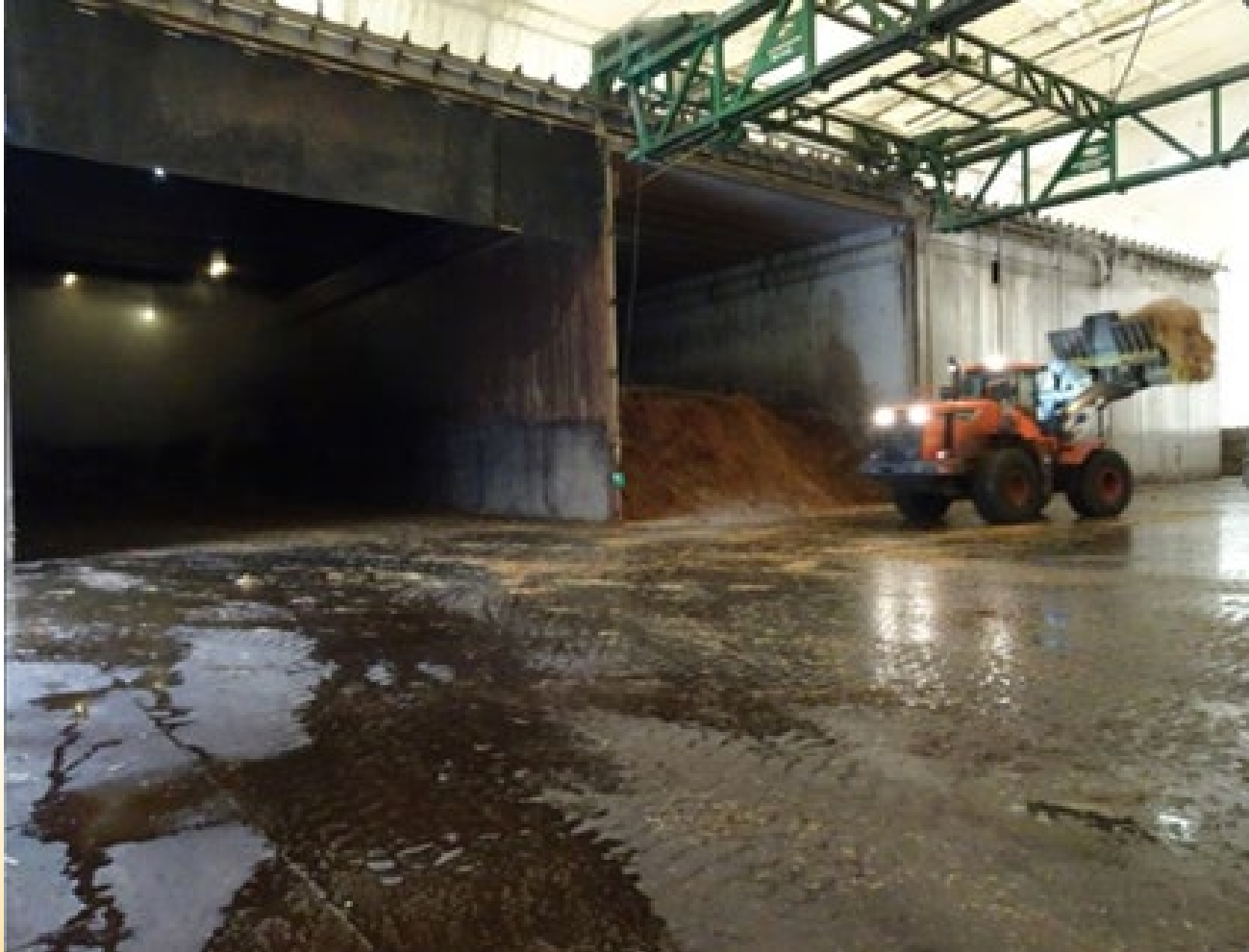
Enclosed Bunker System
