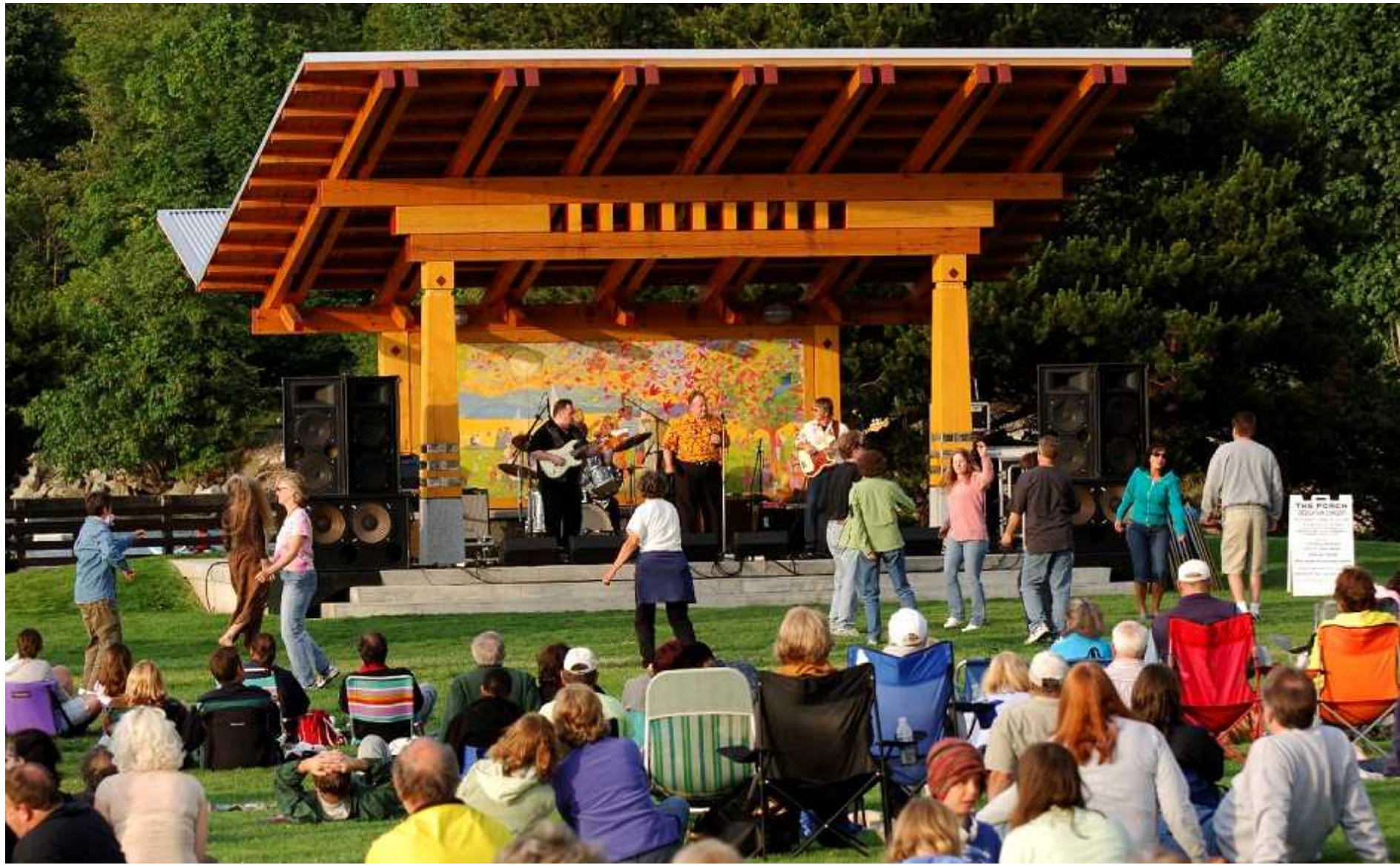
OUTDOOR STAGE/PAVILLION STRUCTURE
